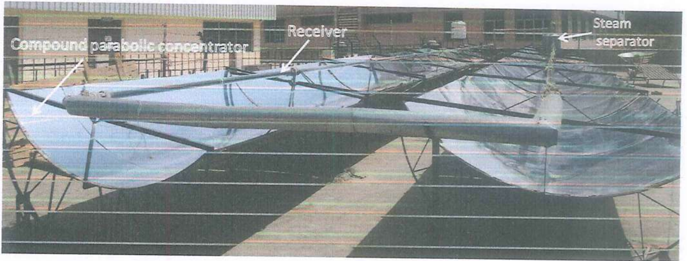
CPC Solar System
